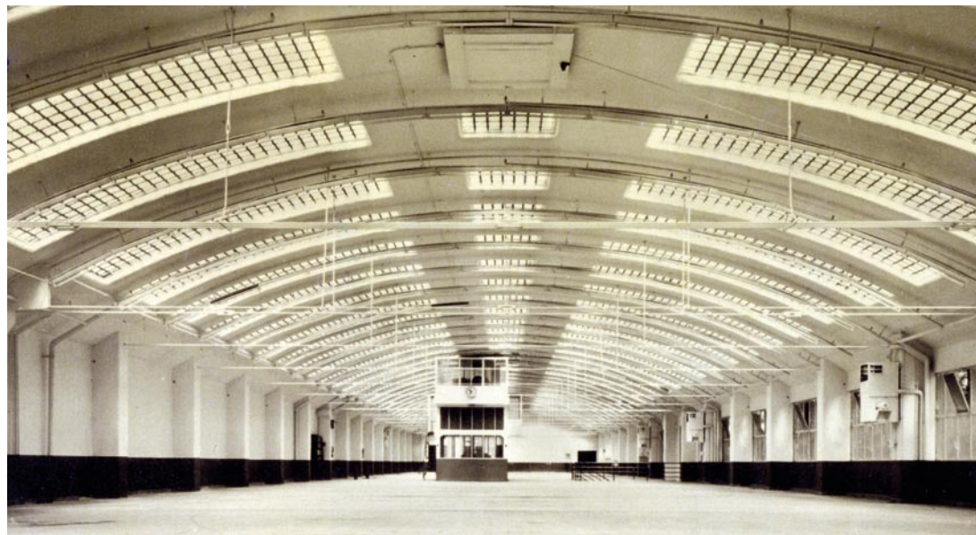
The hall on the new site at Leiersmühle – empty but ready for occupancy.
